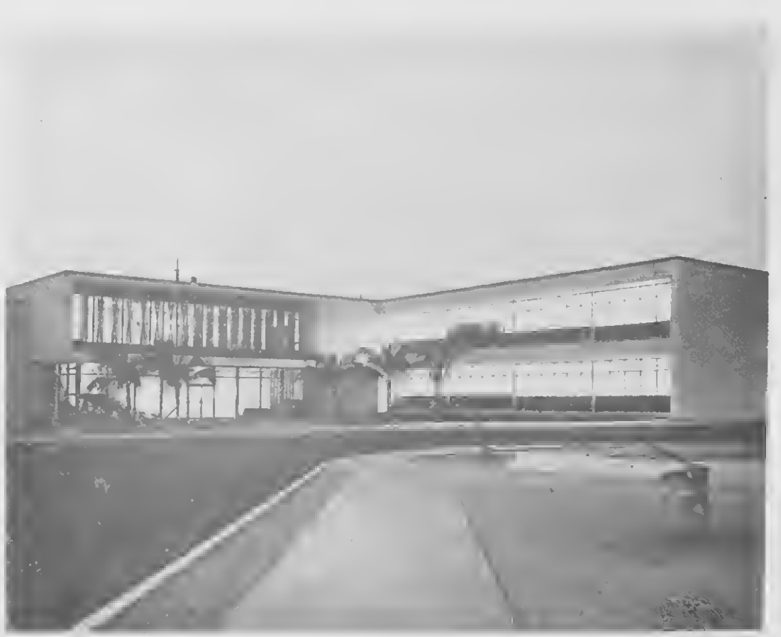
WITH LIGHTS blazing in the early dusk, the new building makes a fine appearance. CU LUZNAN cendí den oranan tempran di atardi, e edificio nobo ta haci un apariencia bunita.
